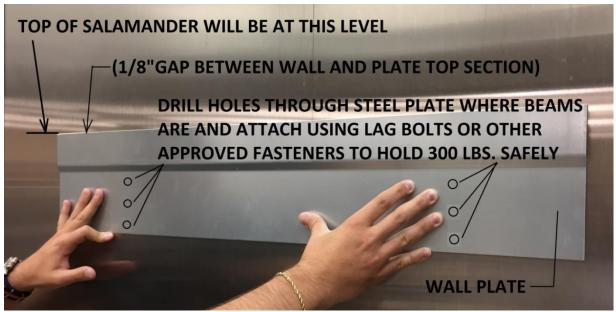
7. After Wall Mounting Plate is secured to wall, lift Salamander (2 people needed) and lower on to wall mounting plate. Plate will extend 2" up in to rear bracket of Salamander. Adjust left and right back leveling bolts to make Salamander plumb and level with wall so drawer is horizontal and level. See drawing below.
